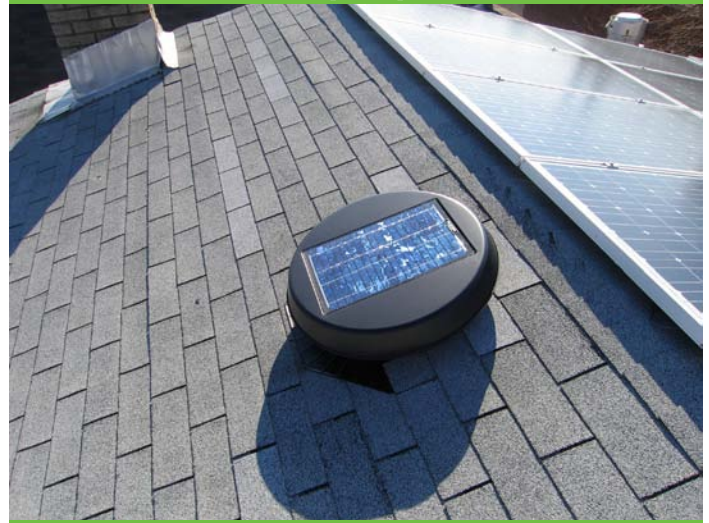
Solar powered attic fan
