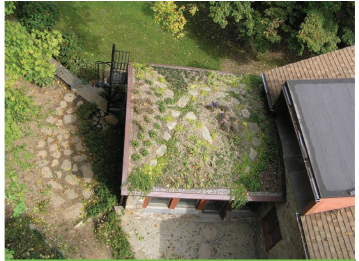
Green roof over new addition
