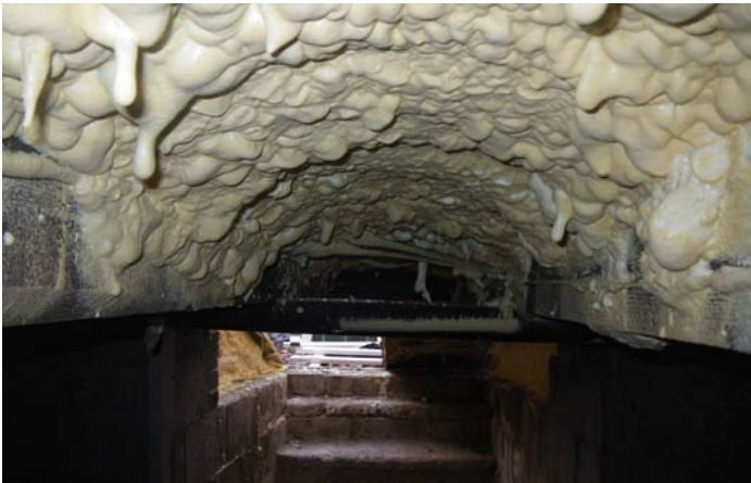
Spray foam insulation in basement (before thermal barrier is added)*
