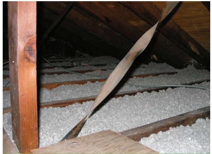
Blown cellulose insulation in attic
