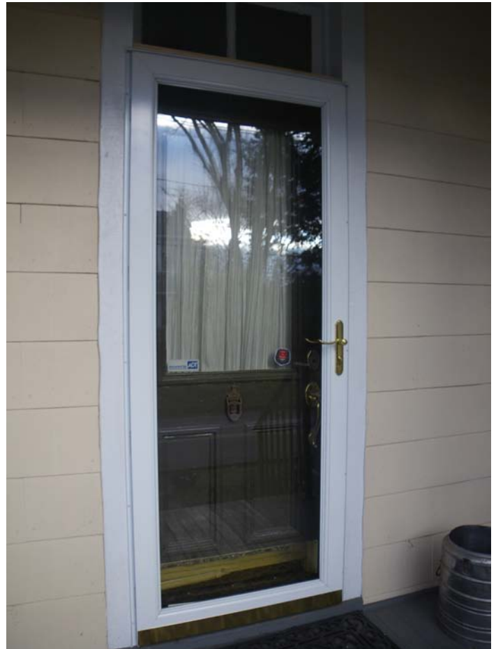
Storm door installed to provide added protection
