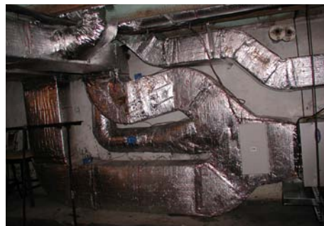
Ductwork sealed and insulated
