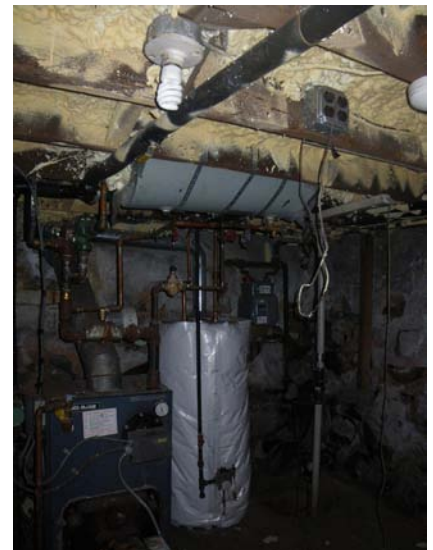
Added insulation in basement (before barrier)*
