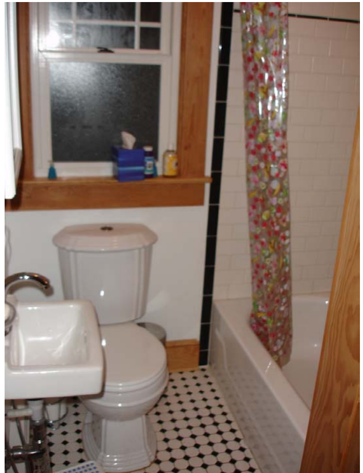
Downstairs bathroom after remodel
