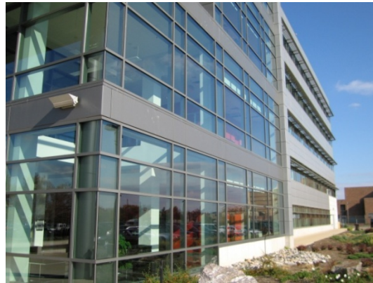
Fig 11: High performance glazing, building envelope. Source: Clinton Andrews
