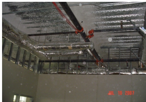
Fig 31: Ceiling space before tenant fit-out Source: Steven Martorana, NJEDA
