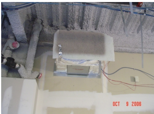
Fig 30: Ductwork sealed during construction Source: Steven Martorana, NJEDA
