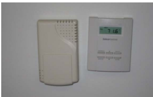
Fig 32: Carbon dioxide sensor and programmable thermostat. Source: Clinton Andrews
