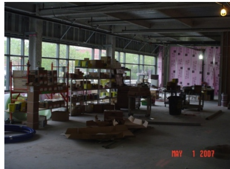
Fig 14: Construction area kept free from debris Source: Steven Martorana, NJEDA
