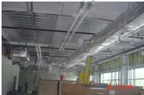
Fig 15: Duct outlets covered during construction Source: Steven Martorana, NJEDA
