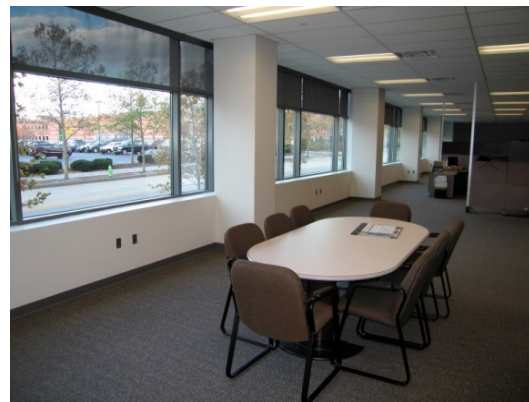
Fig 20: Adjustable interior sun control fabrics in office areas; Source: Clinton Andrews
