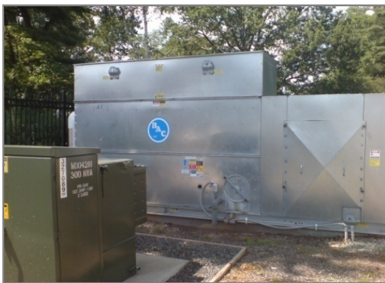
Image 5: Ground-mounted cooling tower. Source: ClintonAndrews
