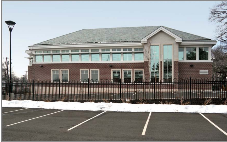
Image 10: Building exterior showing clerestory windows. Source: Image Up Studio, Metuchen, NJ
