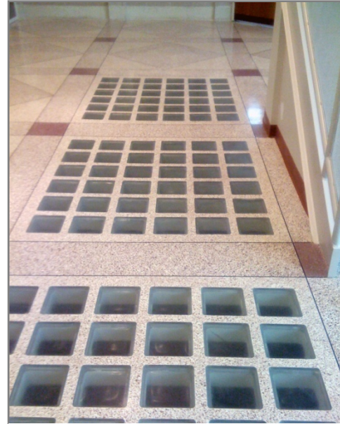
Image 8: Glass tiles in foyer floor allow daylight to penetrate into basement. Source: Clinton Andrews
