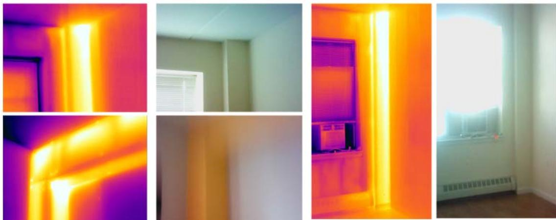
Figure 25. Poorly Insulated Hot Water Risers.
