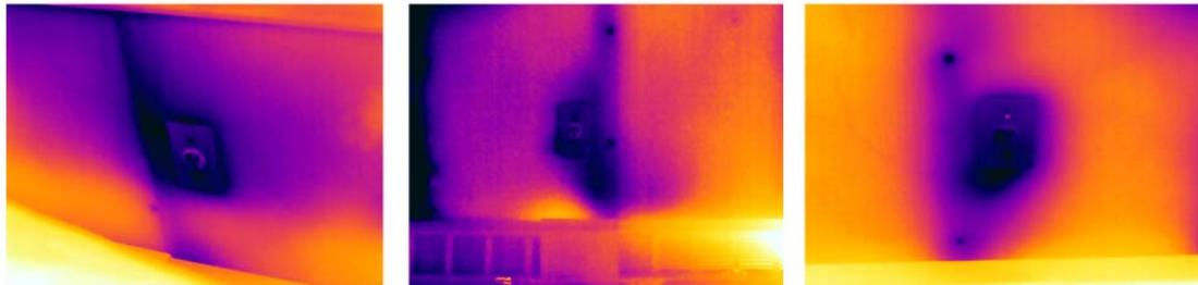
Figure 23. Cold Air Infiltration through Wall Sockets.
