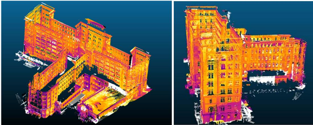
Figure 12. 3D thermal model of building exterior area.
