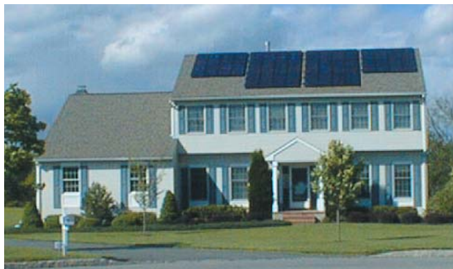
Residential pitched-roof installation in NJ
