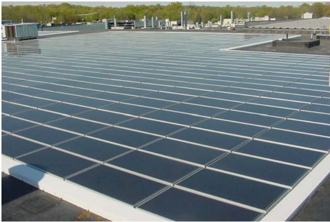
Commercial flat-roof installation in NJ
