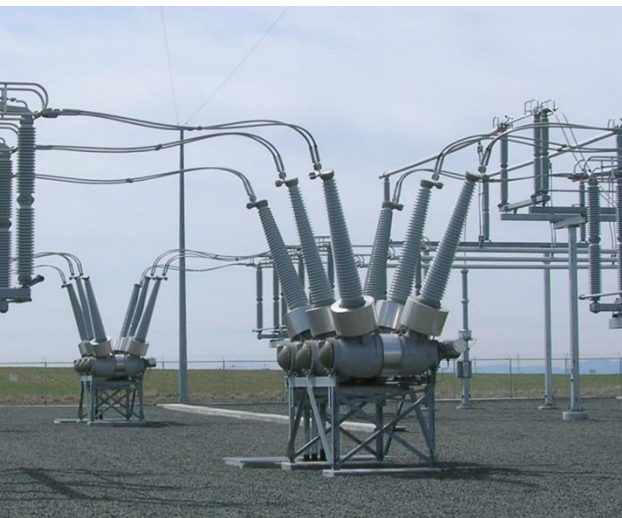
Substation breakers
