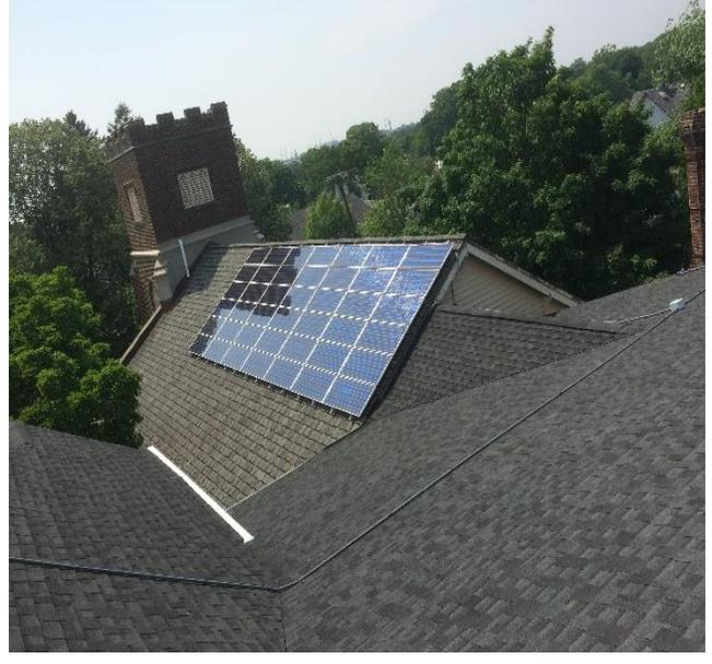
Figure 9: Rack mounted solar panels (42 X 102W) atop one of the 3 buildings at the Reformed Church
