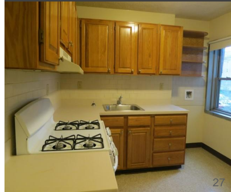
Gas stove at Building M
