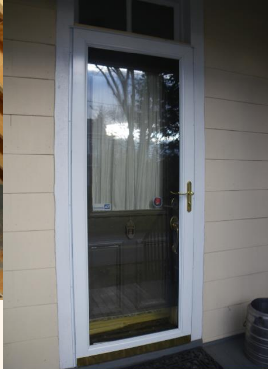
Storm door installed to provide added protection
