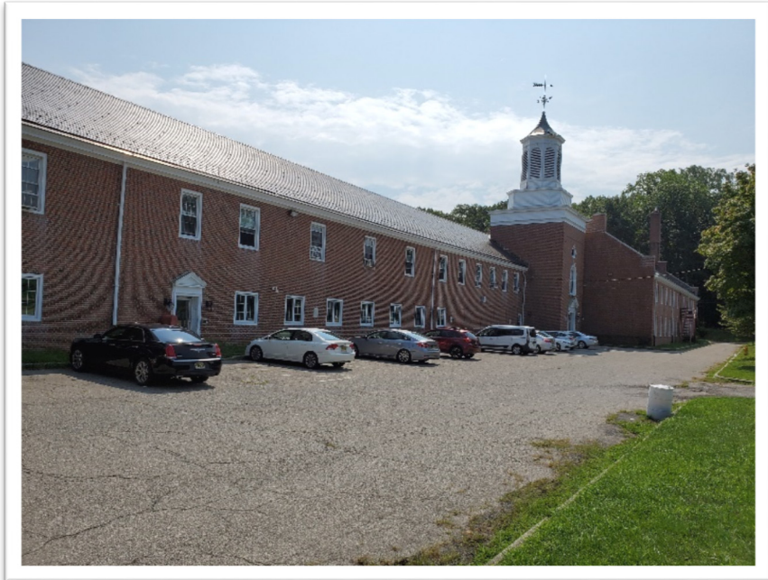
Photo: Building exterior and parking at the Morristown National Guard site.
