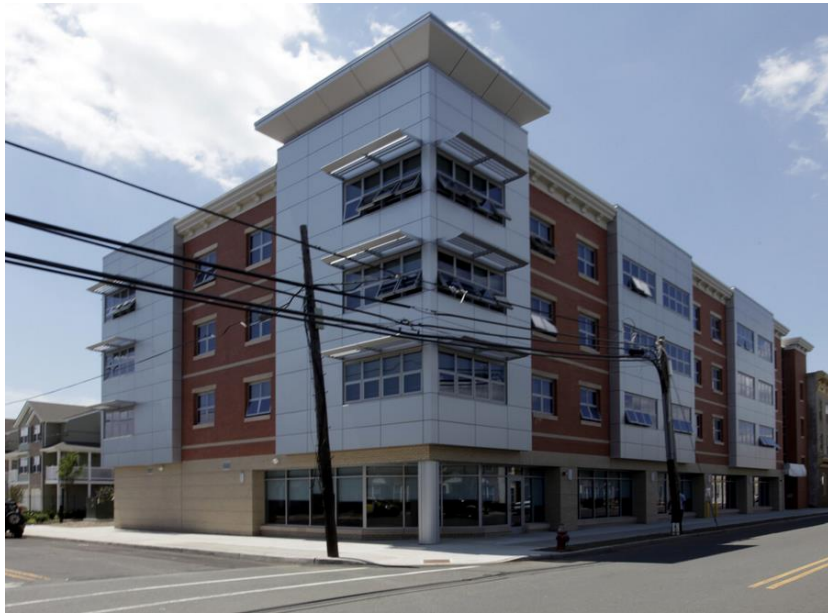
Building Front views and Rear views
