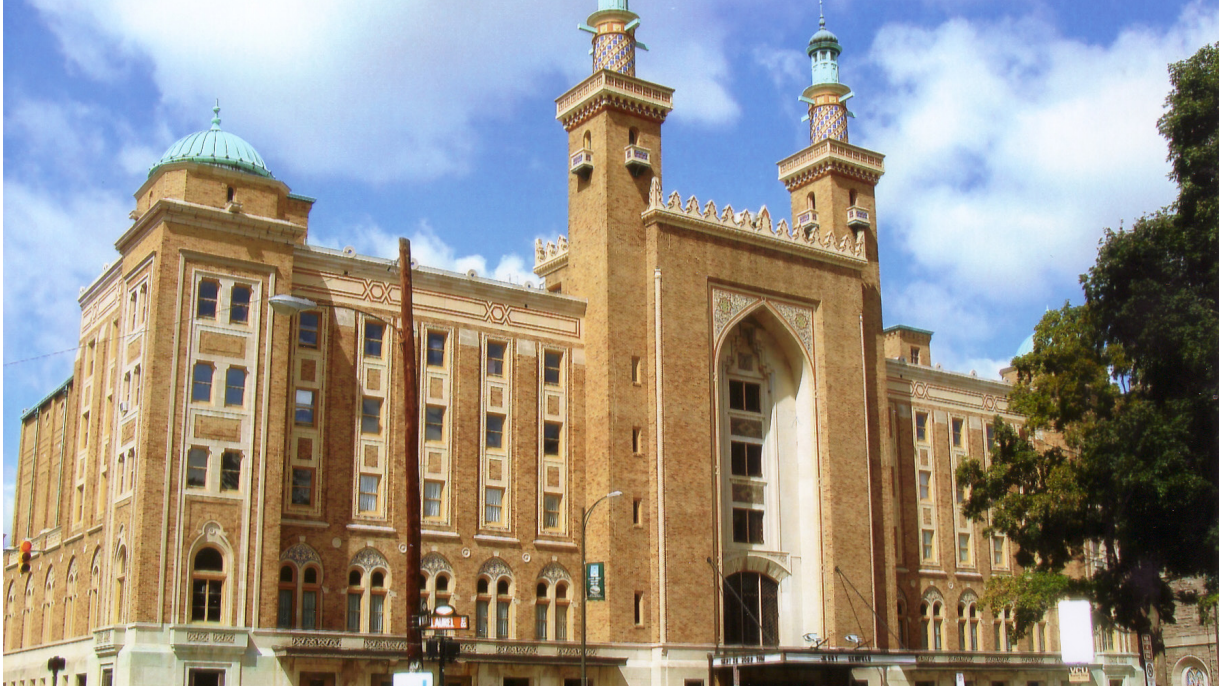
Landmark Theater, Richmond, VA: Originally constructed in 1927, the theater features Moorish Revival design elements and is part of the Monroe Park Historic District. The multi-phase rehabilitation includes repairs to the roof and exterior masonry, building systems upgrades and marquee restoration.
