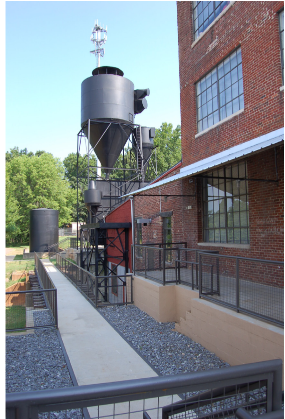
Martinsville Lofts, Martinsville, VA: Built in 1929, this former manufacturing complex was transformed into an affordable residential community of 60 units. The adaptive reuse project features many original elements, such as a Quonset hut and rail spur.
