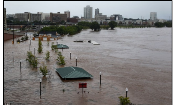
Boyd Park, with inundation caused by Hurricane Irene. 1
