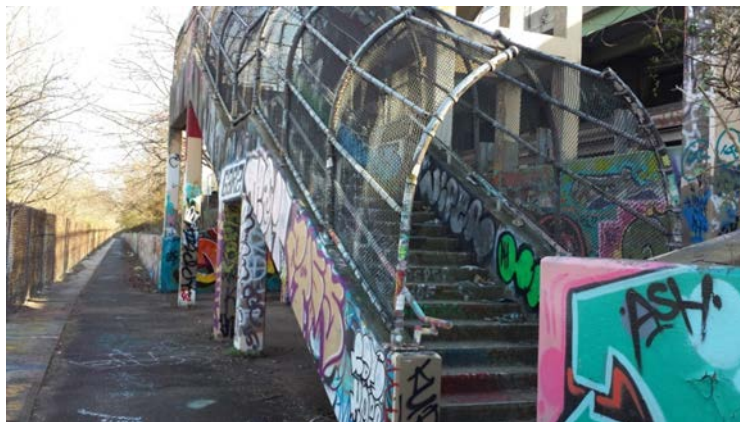
Stairs to the trenchway behind Deiner Park create perception of crime
