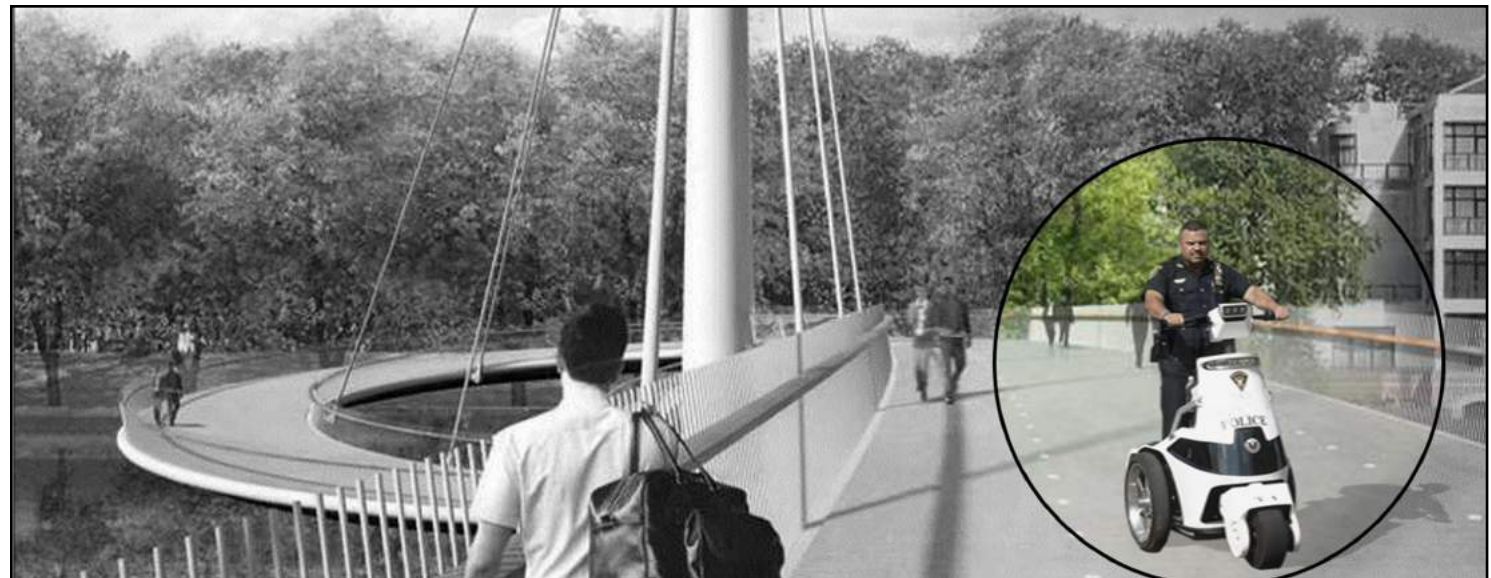
Figure 28: Rendering of required materiality for the bridge and trail to allow emergency vehicle access in both areas.
